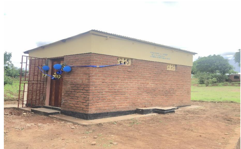
Newly constructed washroom at Chalowe primary school
