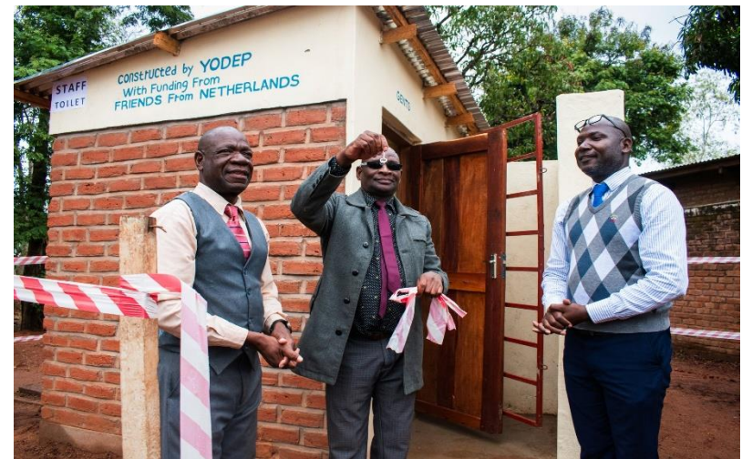
Handover of new toilet blocks at Thundu Primary School
